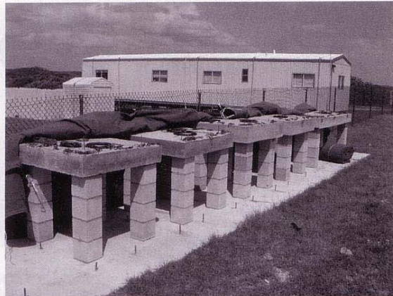
Some of these elevated concrete slabs at KSC's Materials Science Beach Corrosion Test Site have been coated with GLACS to measure the coating's effectiveness in harsh environments.
